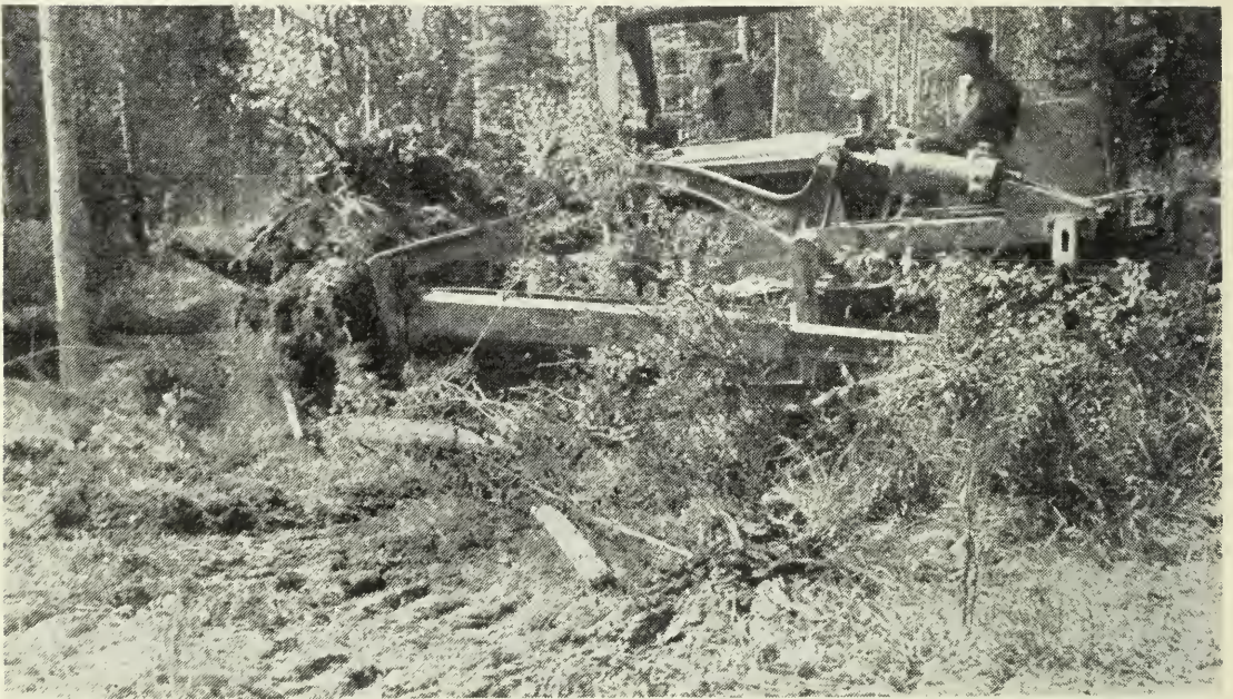
FIG. 8.—Tree, roots, and top soil were removed in one operation.
