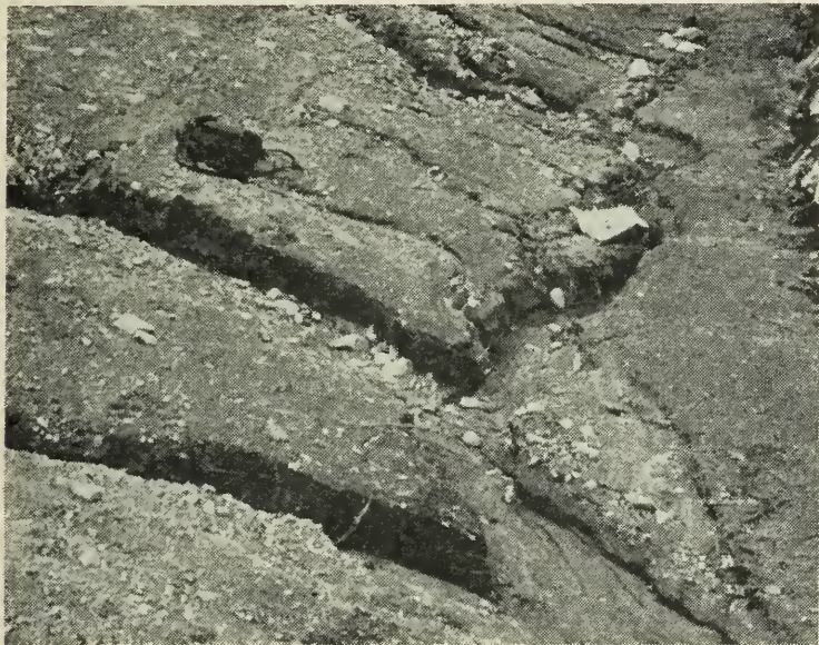
Figure 2. Tailings water from the lower ends of furrows frequently causes serious damage to roadways.
