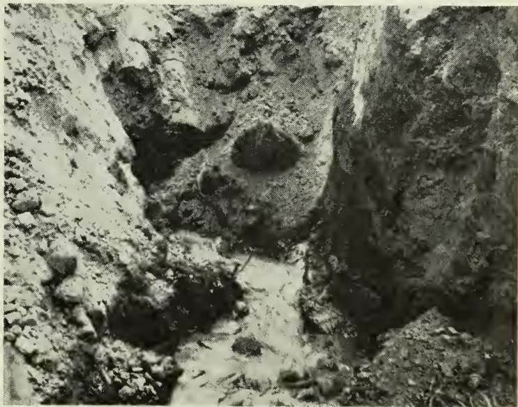
Figure 3. Seepage water emerging from the base of a cliff. In this case, a large section of the hillside collapsed before the spring was brought under control.
