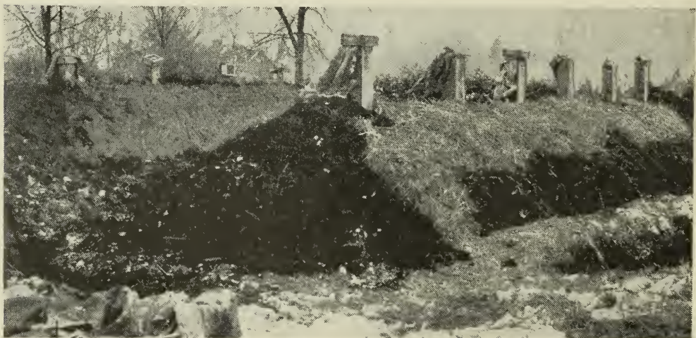
FIG. 9—Root-pit. Final covering of earth and straw being put on. Bags on ventilators for control of temperatures.
