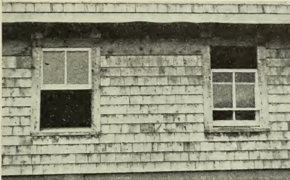
RESTRICTED OR SLOT VENTILATION
