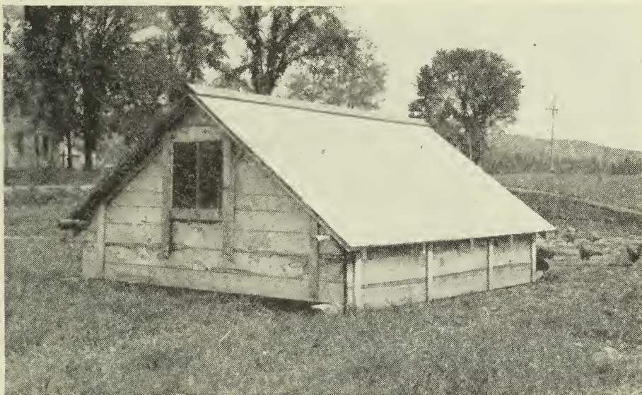
10- BY 12-FOOT RANGE SHELTER
