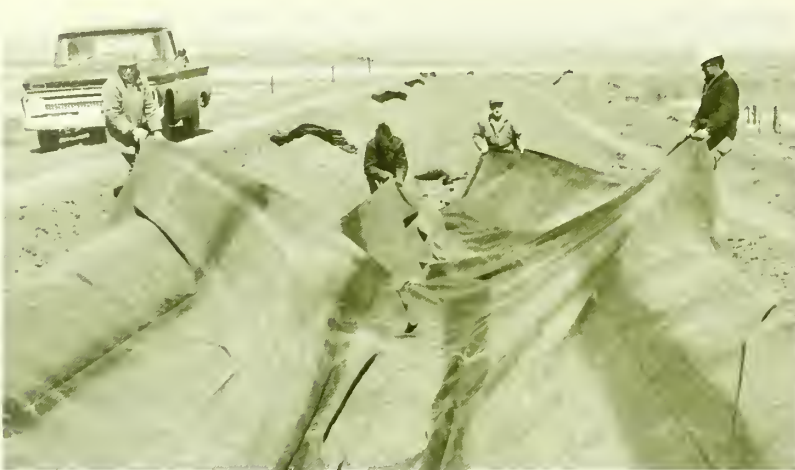
Lining irrigation canal to control seepage.
