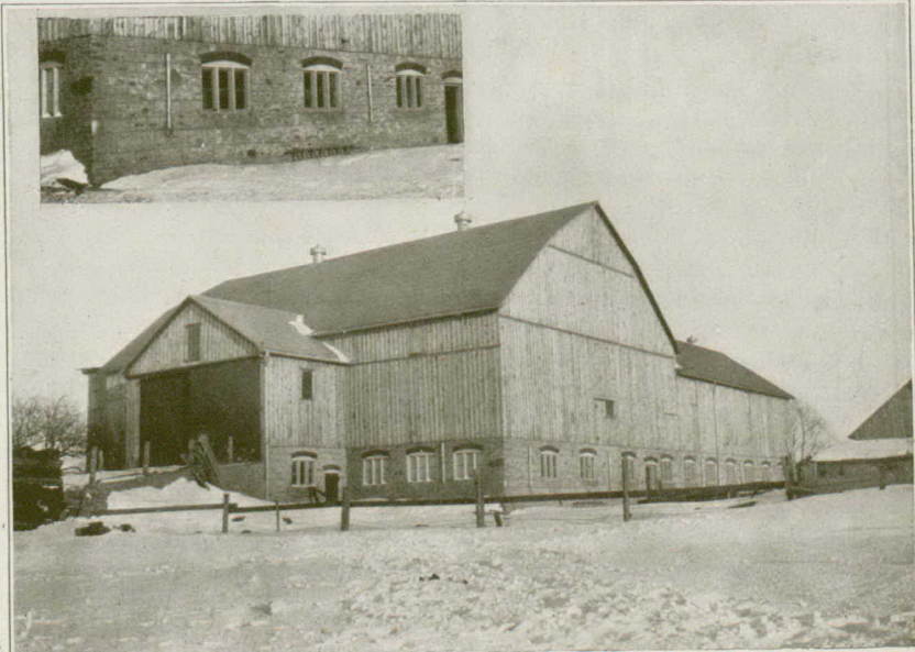
Fig. 65. Barn owned by Biggar Bros., Halton County, Ont. Section at upper corner shows windows, also galvanized metal intake pipes of ventilation system. Interior fittings same as Fig. 64.
