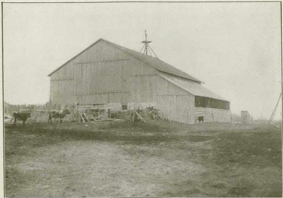
Fig. 50. Deserted Basement Barn, owned by J. L. Cook, Newdale, Man.
