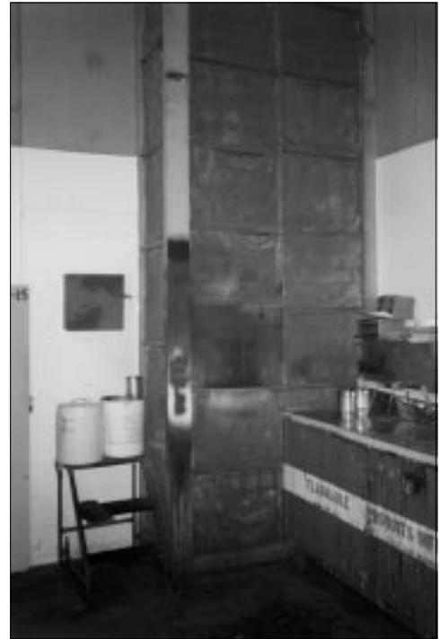
*Dirty and deteriorating dry filters inside a paint booth at Gagetown.*
