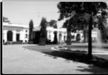
$1.5 million reconstruction of the official residence in New Delhi, India
