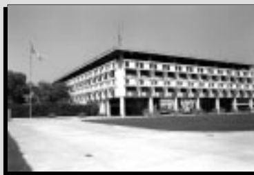
$25.8 million addition to the existing chancery in New Delhi, India
