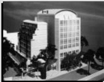
Planned $55.2 million office and residential complex in Seoul, South Korea
