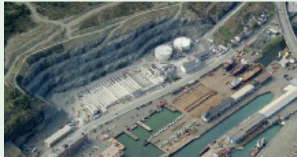
City of St. John's wastewater treatment plant
