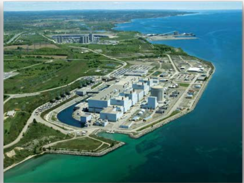
Centrale nucléaire de Darlington (Ontario Power Generation), Clarington, Ontario
