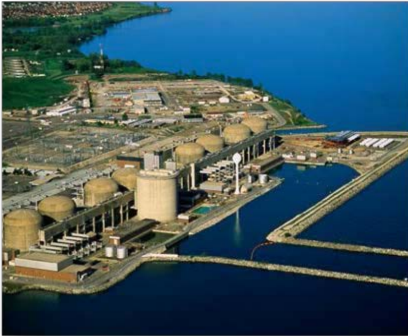
Centrale nucléaire de Pickering (Ontario Power Generation), Pickering, Ontario
