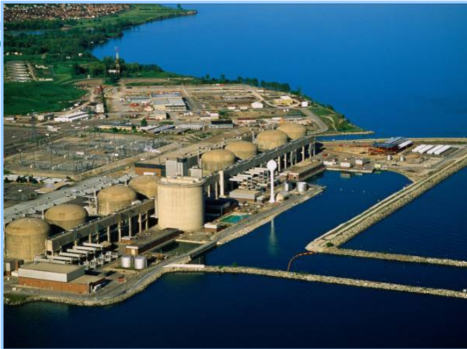
Pickering Nuclear Generating Station (Ontario Power Generation), Pickering, ON
