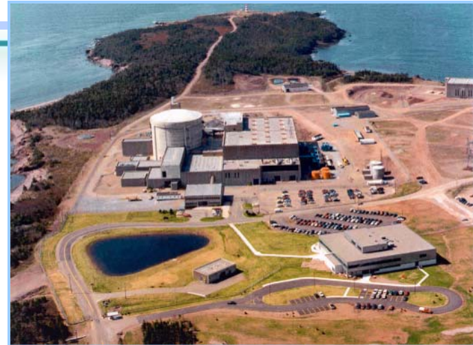
Point Lepreau Generating Station (New Brunswick Power Nuclear), Point Lepreau, NB
