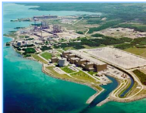
Bruce A and B Nuclear Generating Stations (Bruce Power), Kincardine, ON
