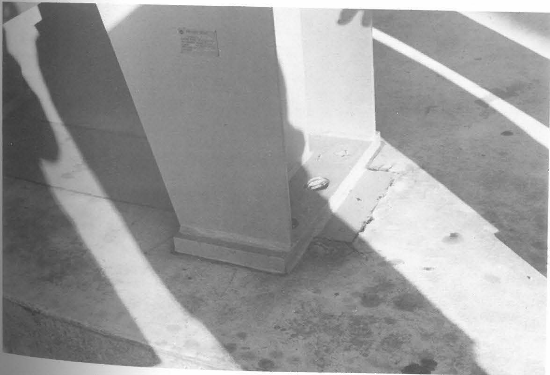
Fig. 5.31 Second generation concept of anchoring device
