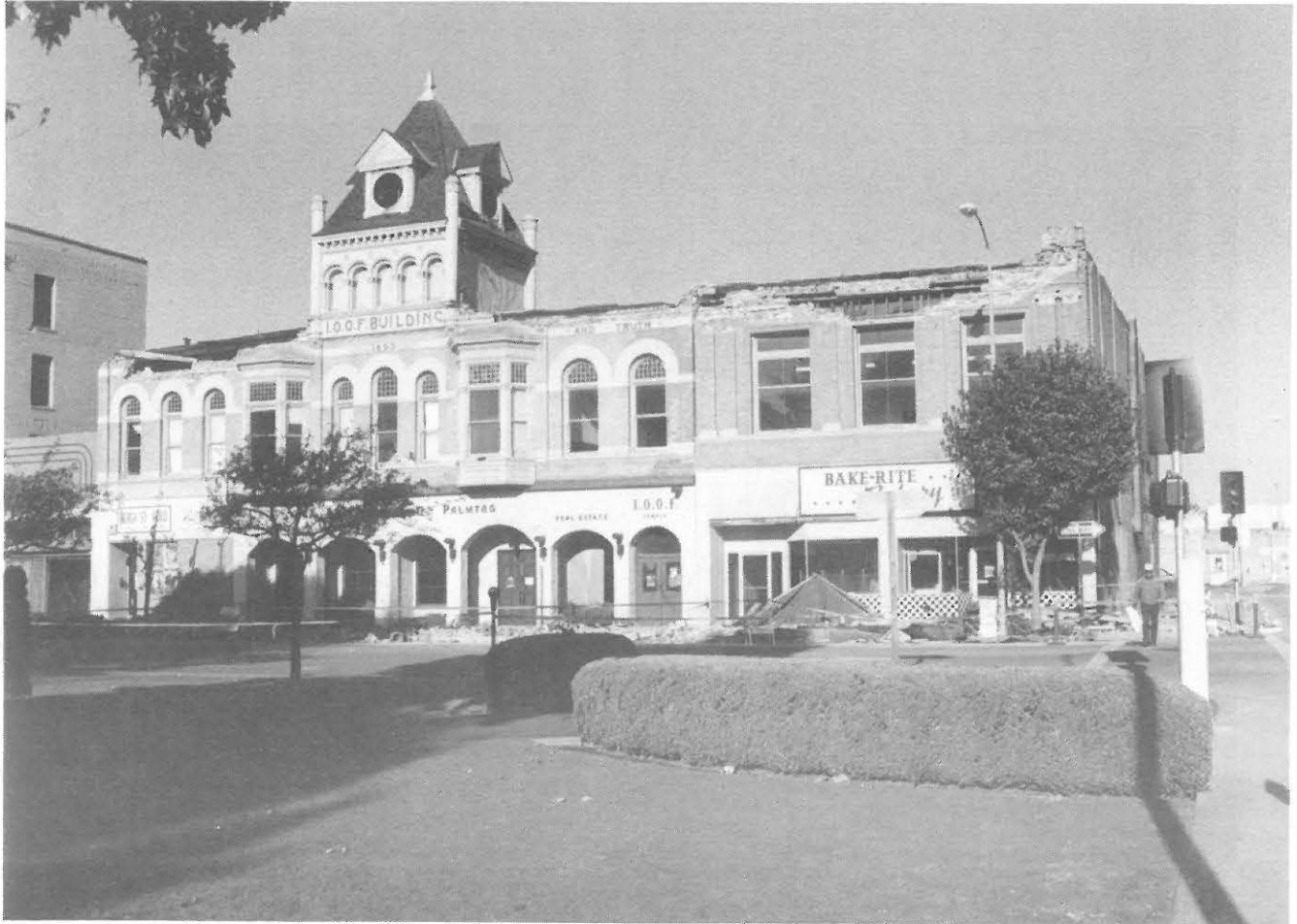
Fig. 3.18. Damage to an old unreinforced masonry building structure - I.O.O.F. Building built in 1893 on East Beach Street in Watsonville
