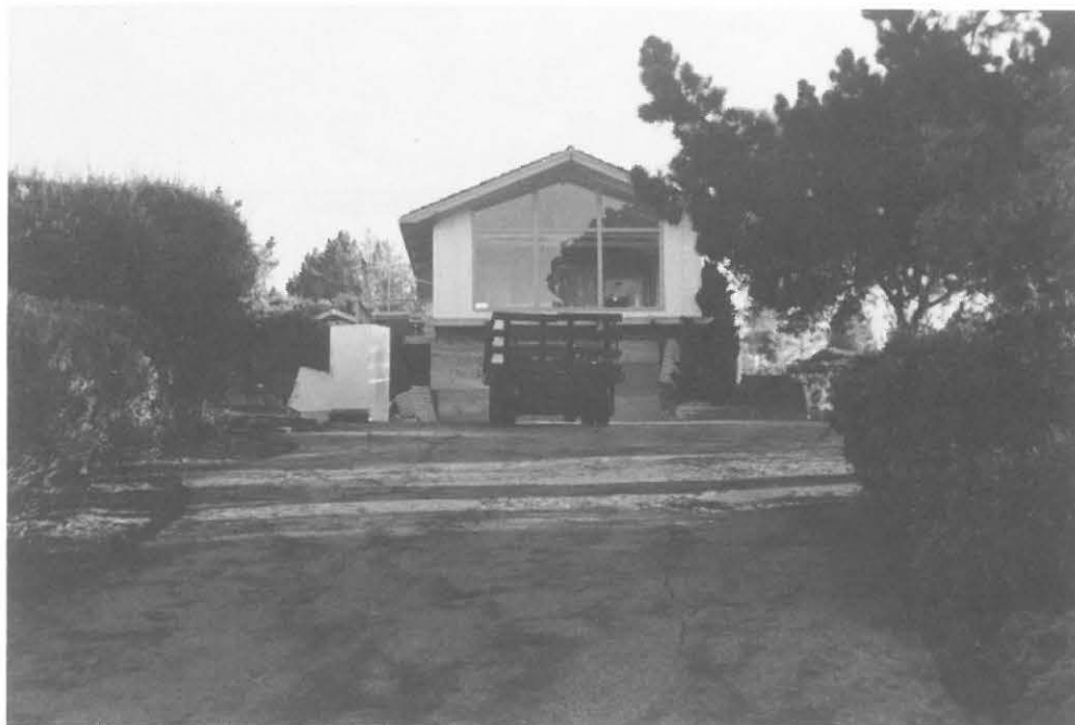
Fig. 3.8 Damage to a modern wood-frame house in Los Altos Hills
