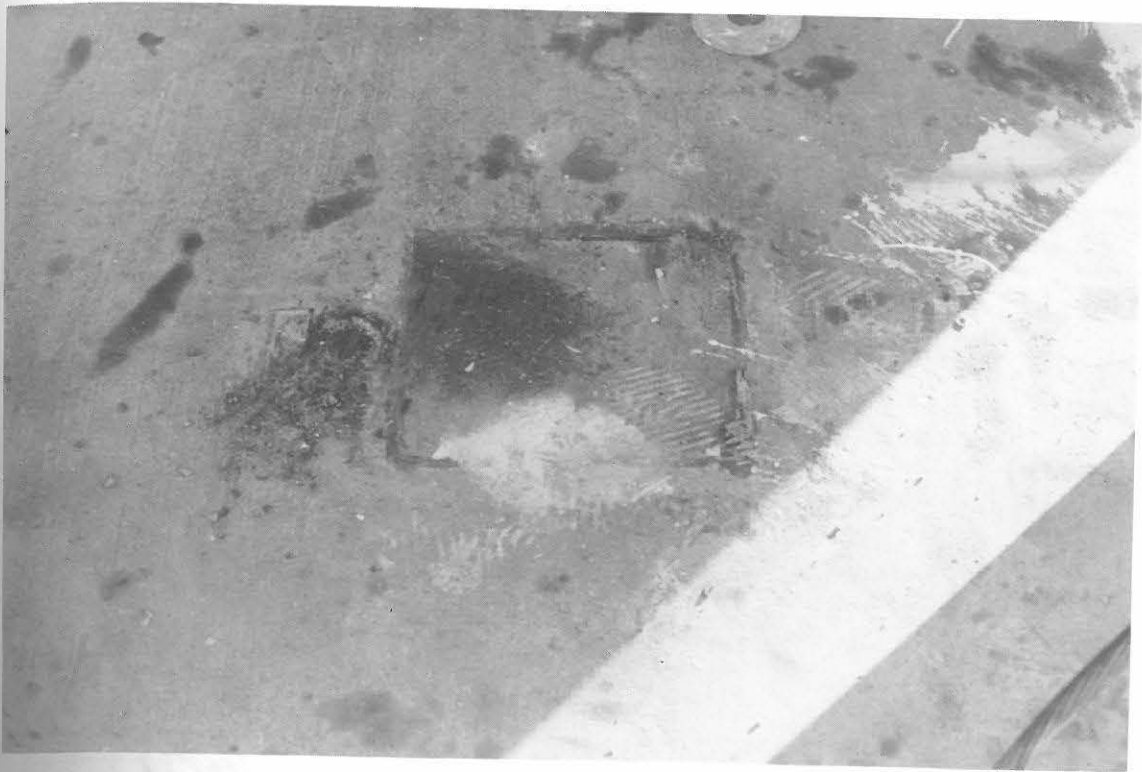
Fig. 5.30 Location of the base plate and of the anchored bolts (an old concept)
