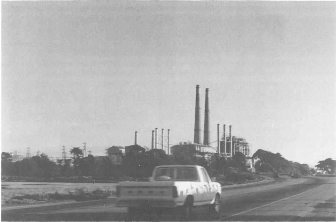
Fig. 5.2 Moss Landing Power Plant
