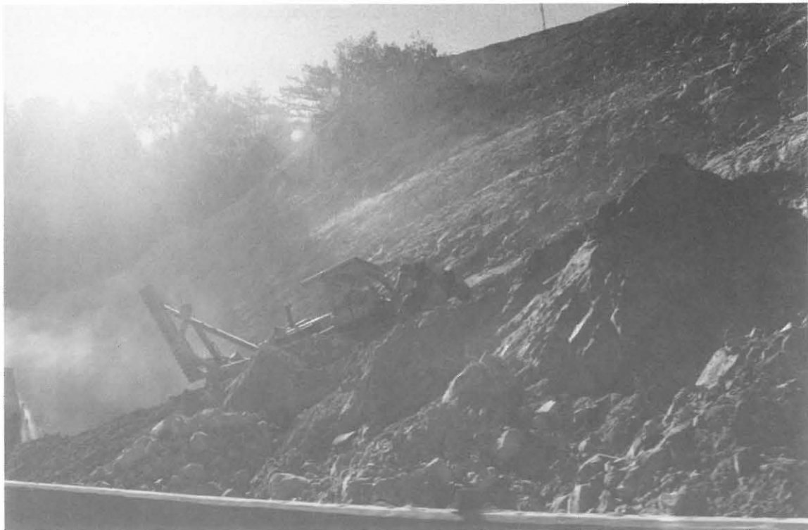
4.20 A dangerous landslide being removed on Highway 17 in the Santa Cruz Mountains
