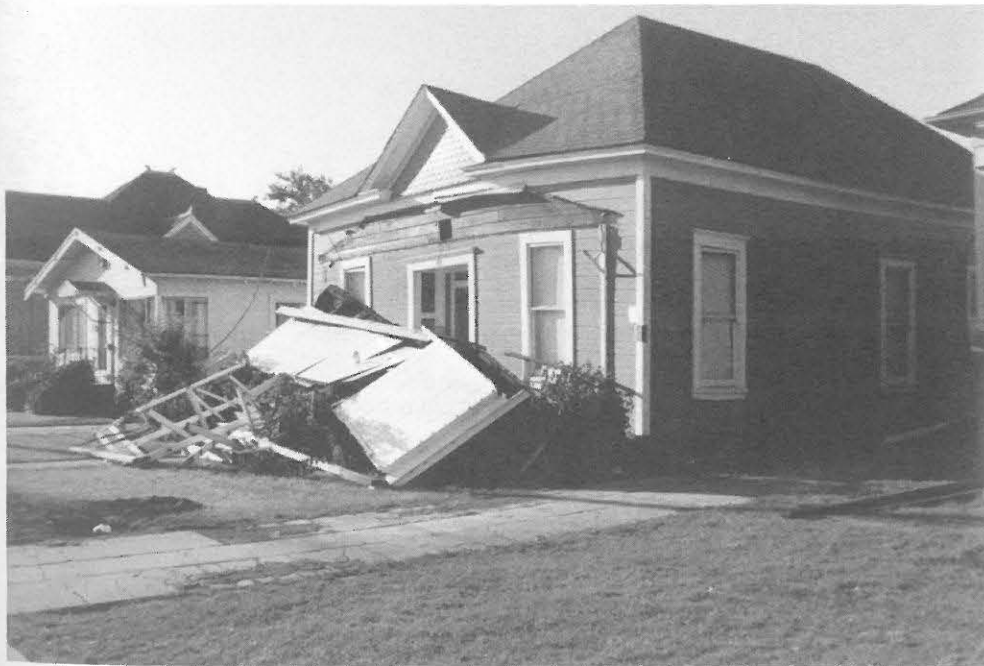
Fig. 3.4 Two houses on Sudden Street, one with cripple wall failure and collapsed entrance porch, and the other with no damage - City of Watsonville
