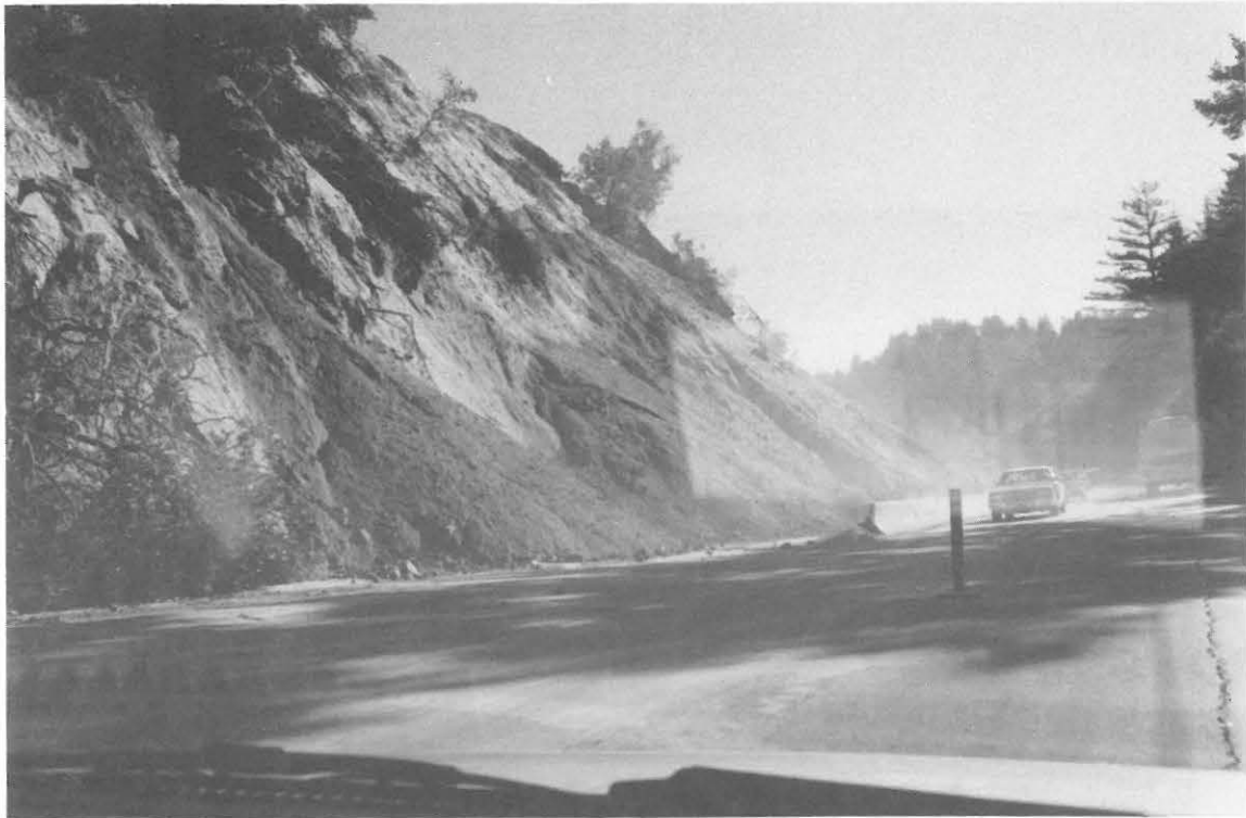
Fig. 4.19 A landslide triggered by the Loma Prieta earthquake on Highway 17 in the Santa Cruz Mountains
