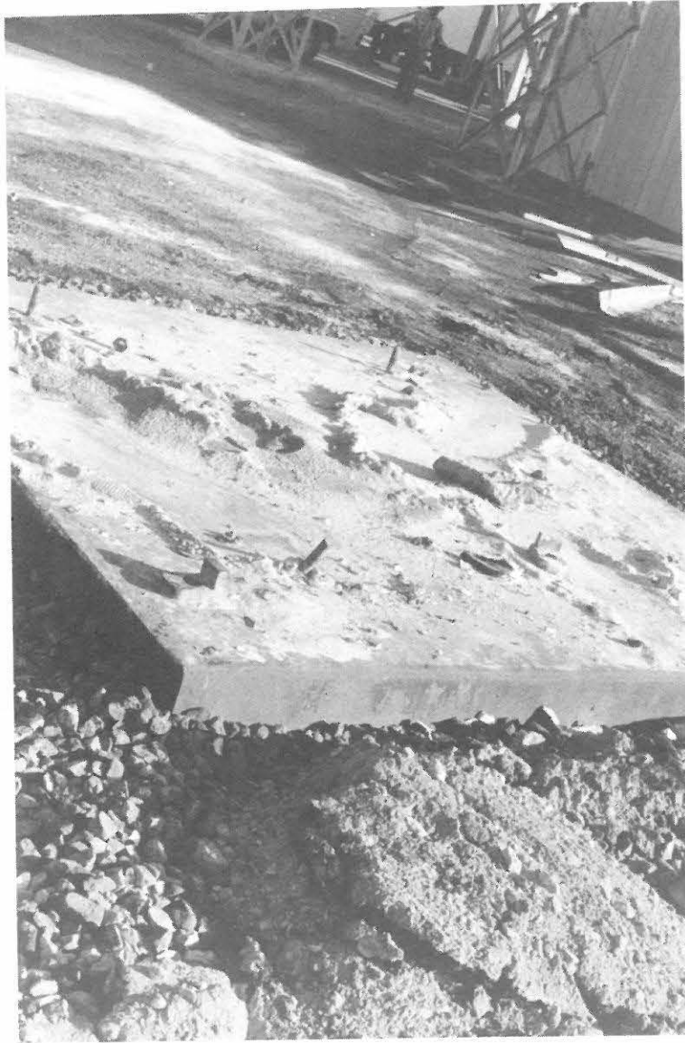
Fig. 5.29 Anchor bolts of the 500-kV SF6 circuit breaker support
