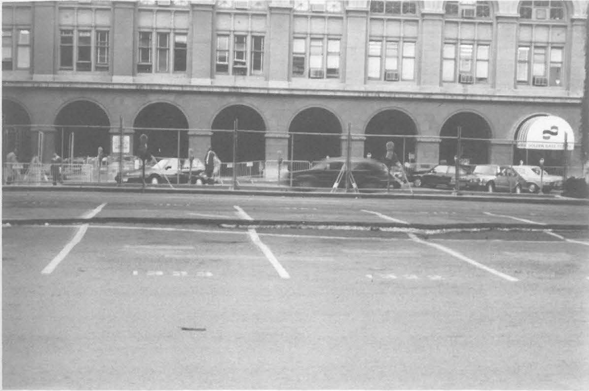
Fig. 2.7 15-cm differential settlement under the Embarcadero Freeway
