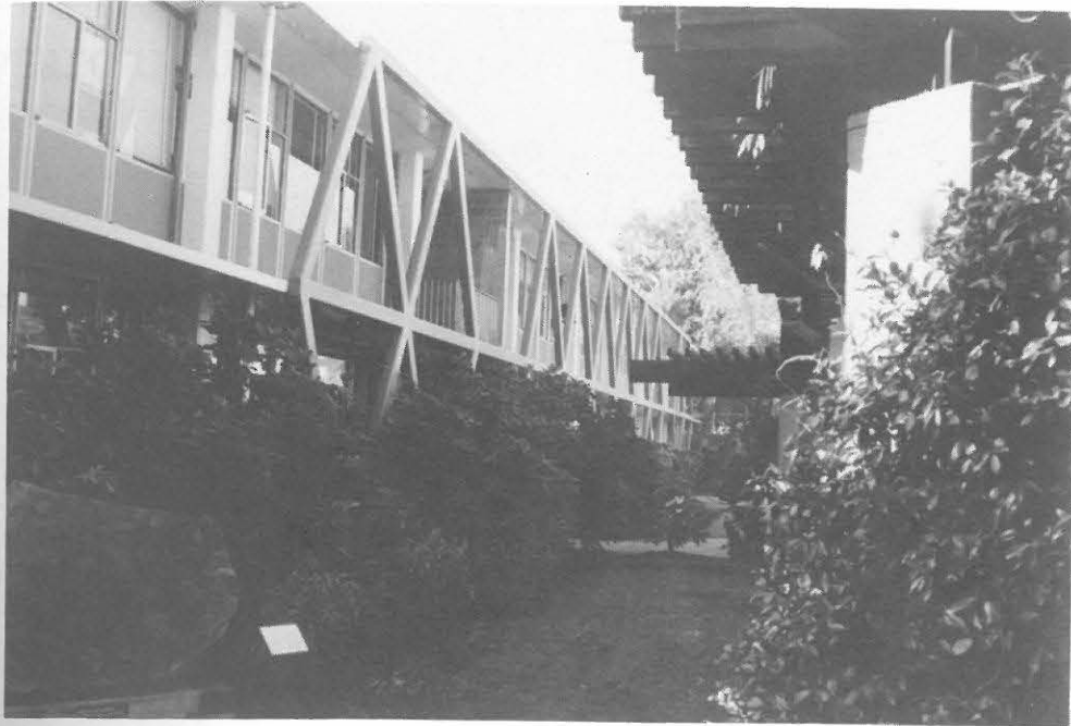
Fig. 3.26. Seismically upgraded concrete-frame building of the U.S. Geological Survey in Menlo Park, California
