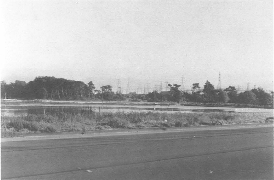
Fig. 5.25 View of the substation and power generating plant sites at Moss Landing Power Plant
