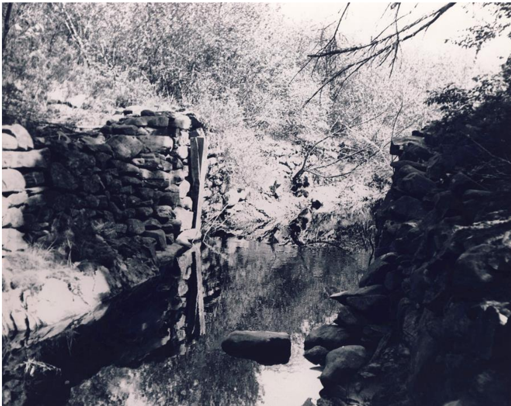
Figure AI-2: Stone control structure in the Sand Pond canal circa 1965 Photo: © Environment Canada
