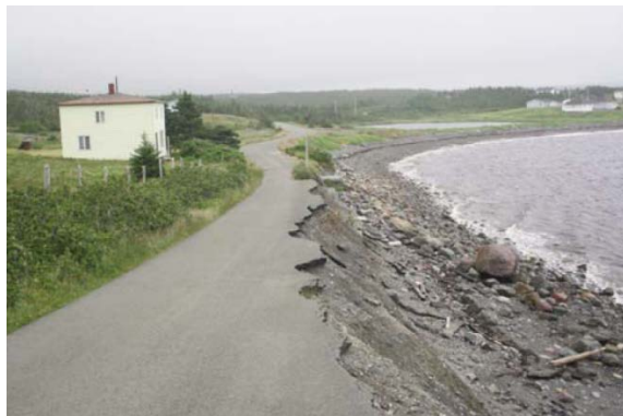
Figure 32. Coastal erosion at Admiral's Beach, Avalon Peninsula, undercut this transportation route. Source: Batterson and Liverman, 2010 181
