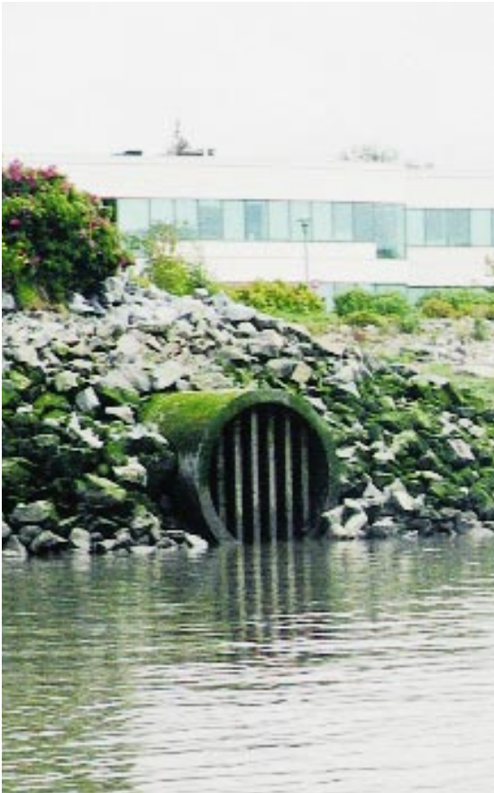
Greater Vancouver is gradually phasing out obsolete storm drain technology.
