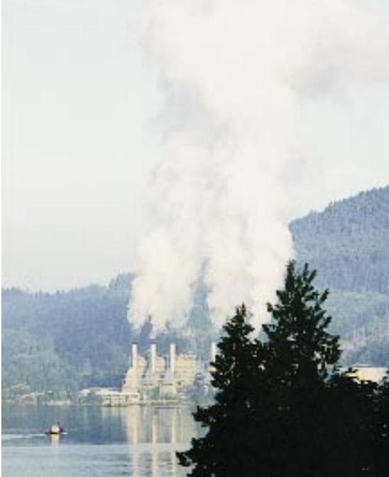
A thermal power station
