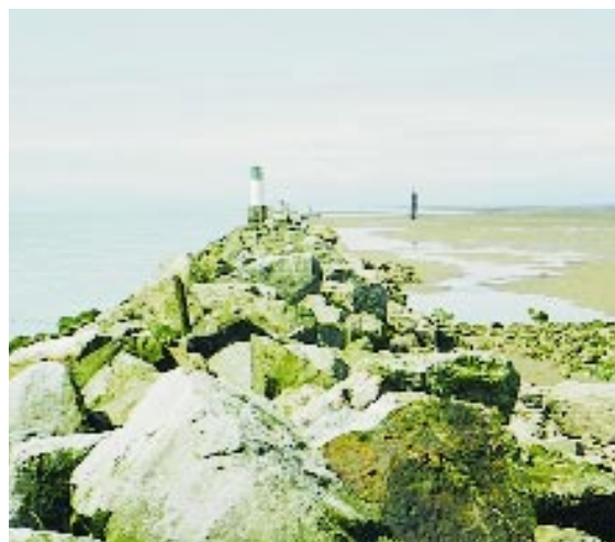
A jetty keeps tidal flats from being naturally replenished with sediment.
