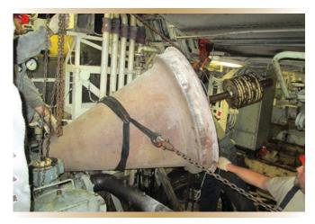
Figure 4. Removing the diffuser cone.
