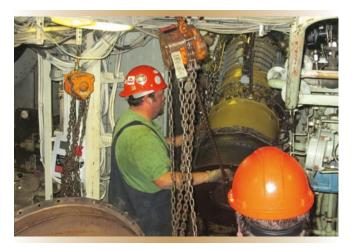
Figure 8. The new engine is eased carefully into the enclosure.
