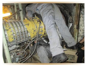
Figure 9. Allison Gas Turbines FSR Russ Brown ensured the alignment between the engine output and the gearbox was absolutely straight.
