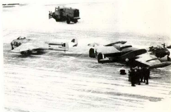
Removing ice with a jet blast
