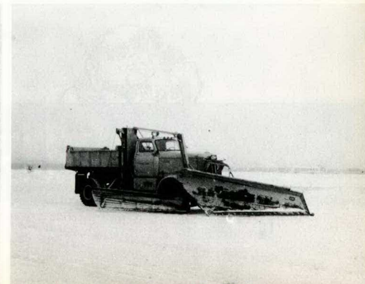
One-way plow with levelling wing
