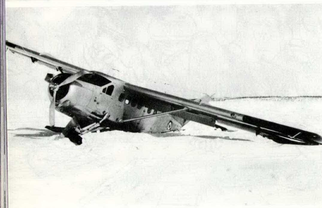
The pilot pulled off early and had a wing stall.
