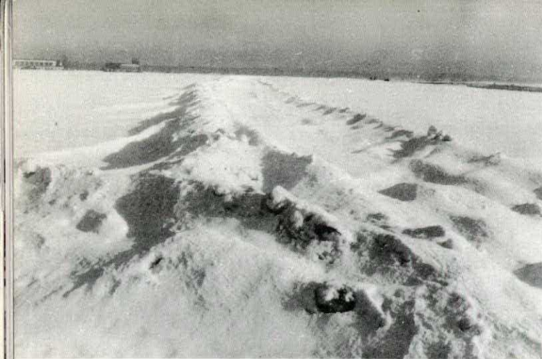
Snowbanks ploughed parallel to one side of a runway will prevent snow from drifting across its surface.
