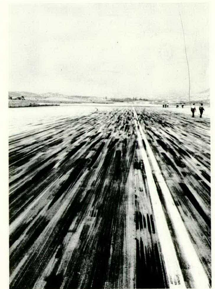
Heavy black marks at the approach end of your runway are proof of premature touchdown.
