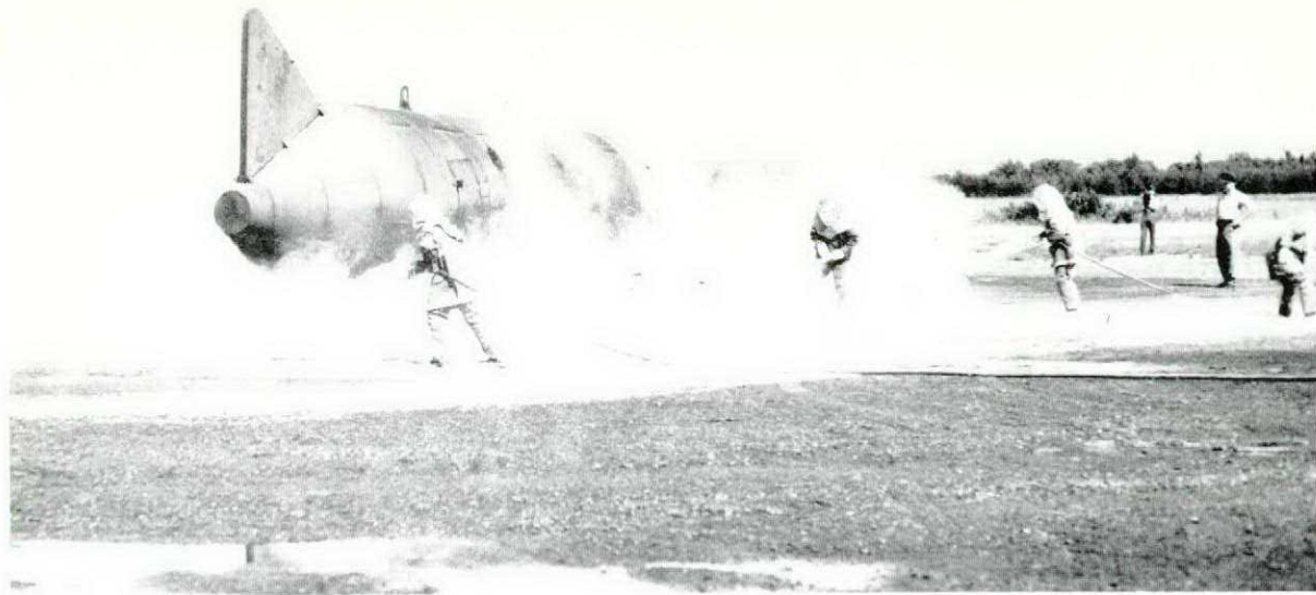
G13 Crash Truck (LRV). Clouds of dry chemical are dispensed. Three handlines are shown, one from a second truck. The mockup aircraft is a training aid at the RCAF firefighter school.
