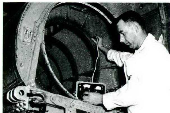
Eddy current conductivity check for strength reduction on aging structure - a CF100 tunnel liner.
