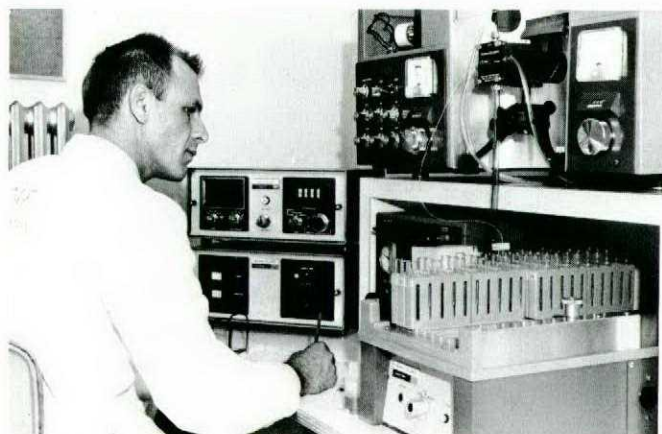
Technician at the AMDU spectrometric oil analysis laboratory runs all samples through an atomic absorption spectrometer. This machine can measure traces of metal in the oil down to parts per million; abnormal rates of increase in metal contamination of an engine's lubricants alerts technicians to possible trouble.
