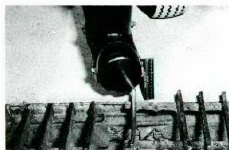
Any "known hazards" around your hangar?
