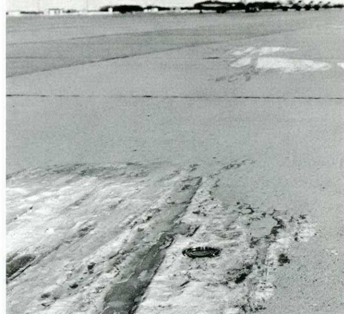
Lid laying in wait
