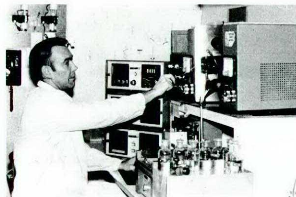
OIL ANALYZED BY SPECTROMETER. MCpl AR Dalglish of the Non-destructive testing centre. The Spectrometric Oil Analysis Program (SOAP) measures the metallic content of aircraft engines oil.
