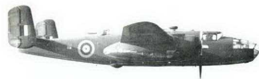
National Aeronautical Collection example of "hard nosed" Mitchell. This nose was sometimes modified to provide for the mounting of eight forward firing fifty calibre machine guns. American Units in the South Pacific mounted a 75 millimetre cannon in some aircraft used in the anti shipping role. Apparently it was quite impressive in effect.
