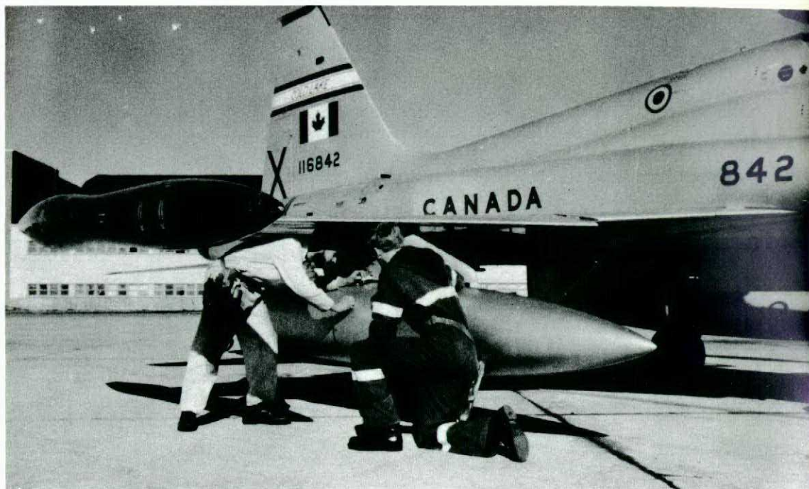
The experimental coverall, complete with reflective tape, hood, and front zipper closure. It was tested with a one-piece insulated underwear, and will be included in the coverall review.
