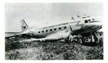
After landing, the aircraft commenced a swing to port which the pilot failed to check correctly. The result - another aircraft damaged extensively and categorized as "B".
