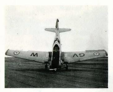
A student pilot was being given a circuit check. After touchdown the Harvard swung to port. The student took corrective action but the instructor overrode his control. without informing the student, and applied harsh starboard brake. The aircraft then developed a swing to starboard and it seems both pilots applied harsh port brake which caused the Harvard to flip up on its nose. This is the old story of neither pilot knowing who had con-
