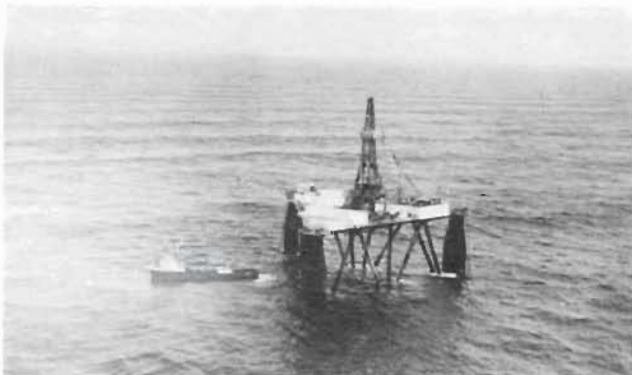
FIG. 6.7. Westerly swell at Shell exploratory drill rig 35 km west of Esvevan Point, Pacific coast Vancouver Island, December 1968. Vessel about 61 m (200 ft) long and distance between vertical supports approximately 85 m (280 ft). Swells have wavelengths about 60–100 m and heights 2–3 m. (Courtesy R. H. Herlinveaux)
