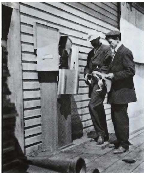
Figure 4. Dr. Dawson (left) and H.W. Jones Inspecting Port Alberni Tide Station, 1909
