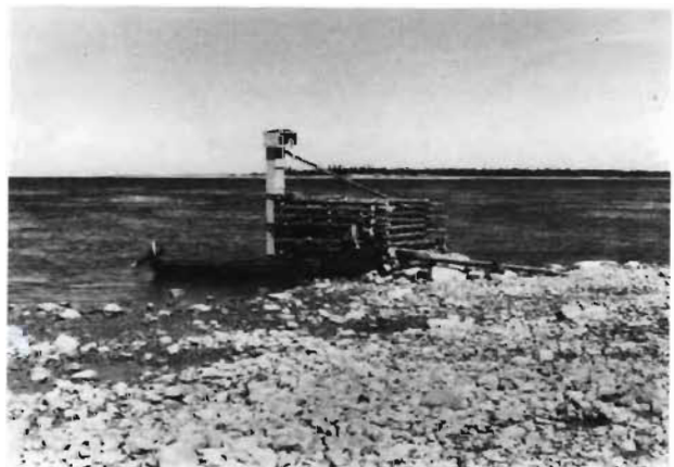
Figure 11. Crib Constructed for Float Gauge, Eastmain River, James Bay, 1958
