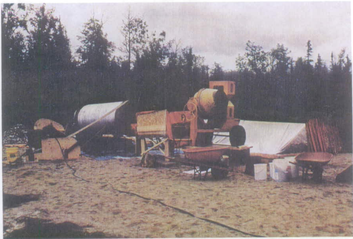
Figure 11: Rockwasher test site
