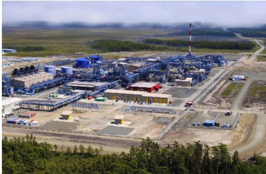
Figure 4-4: Example of an Oil/Gas Treatment Facility (Ref. /34/)
