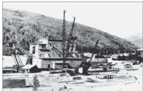
Dredge No. 4 operating on Bonanza Creek
