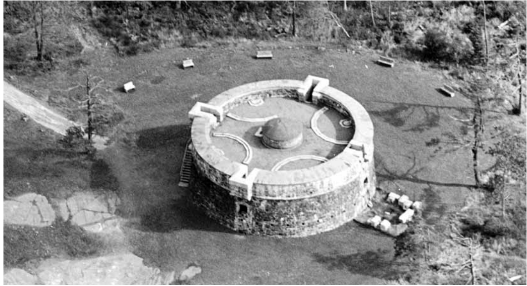
Aerial view of Prince of Wales Tower. Ship to Shore Photography/Parks Canada 2005
