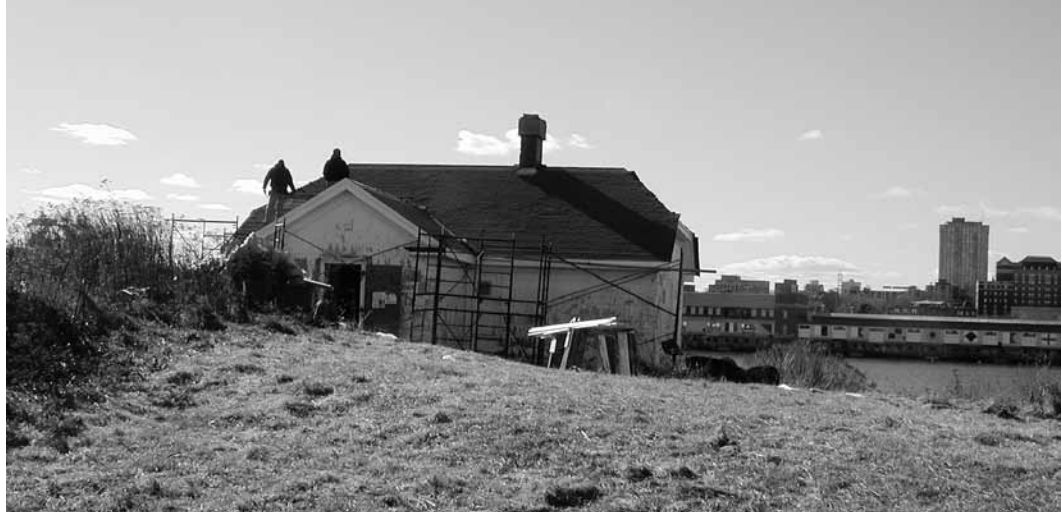
Repair of lightkeepers building, Georges Island. Soonya Quon 2005
