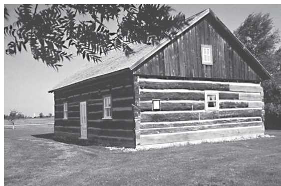
Log house built using the "pièce-sur-pièce" construction technique Parks Canada / Sophie Grenier
