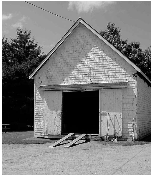
Barn/Carriage house. Parks Canada, 2001
