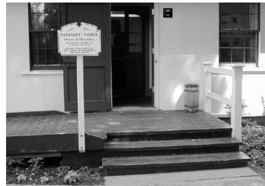
Side entrance to house with signage. Parks Canada, 2001
