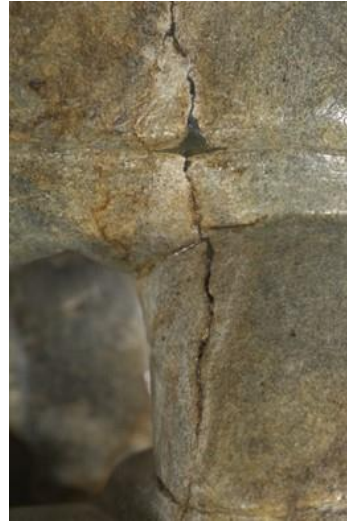
© Government of Canada, Canadian Conservation Institute. CCI 99195-0007 Figure 6. Fill material (probably epoxy resin) was used to fill an area of loss in the stone.
