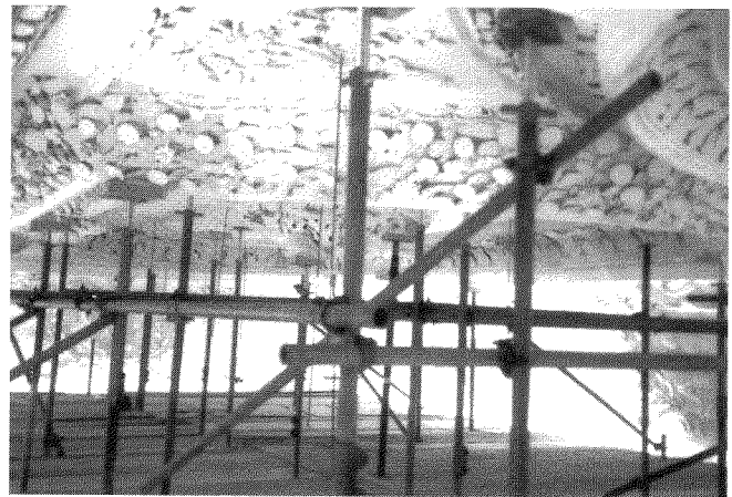
Figure 3. Propping system in place prior to work commencing. Photo: Chris Daniels.
