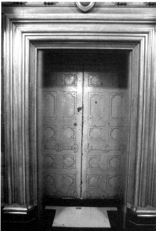
Figure 3. Fire doors to the Library of Parliament which date prior to 1916.
