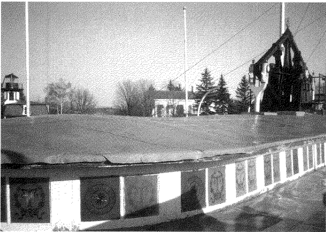
Figure 5. Turtle dome windows and deck with aluminum roofing flashing, 1993.
