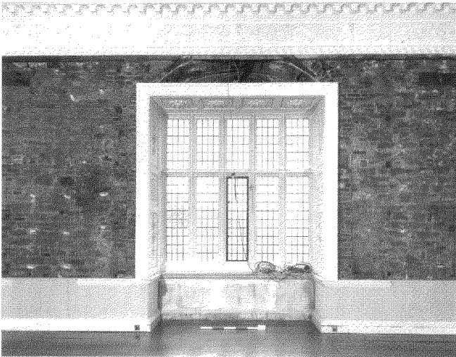
Figure 8. The north wall central window bay with its restored stonework.
