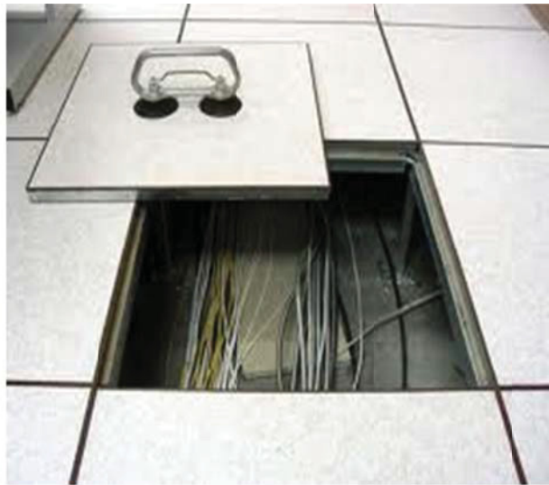
Figure 72: A typical raised floor system.
