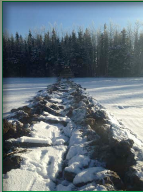
Figure 2a. First pass of an overlapping pass of a winged subsoiler on a bulldozer
