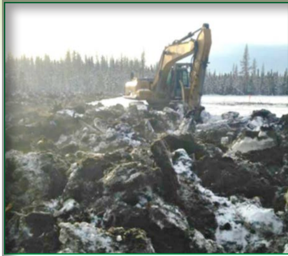
Figure 7a. Rough and loose soil treatment with an excavator and bucket
