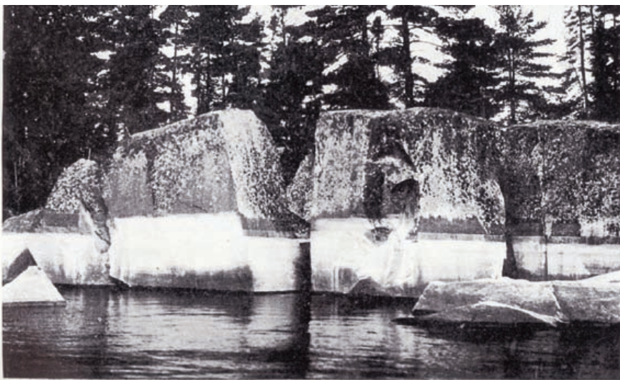
Figure 12 - Distinct high water marks at Rainy Lake, ON (1915)
