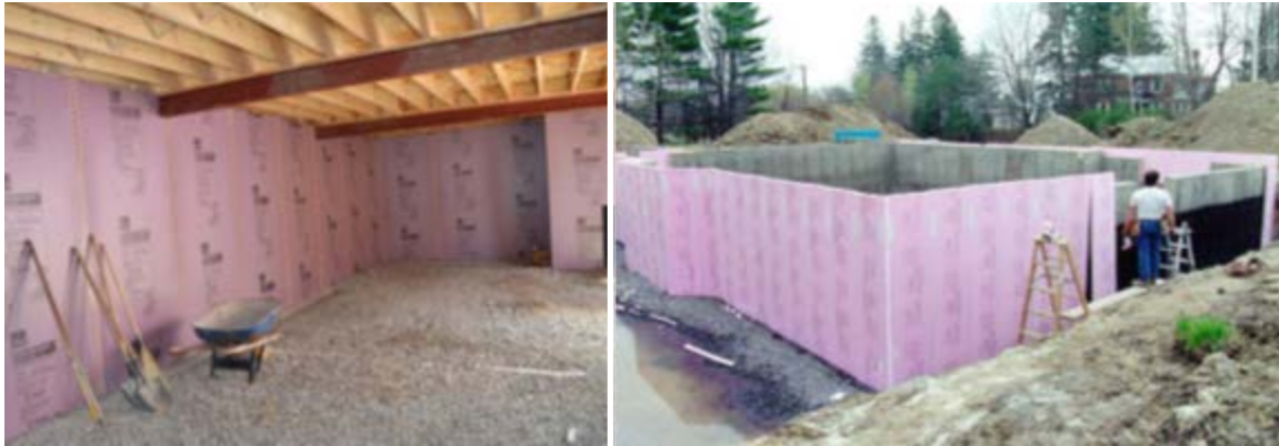
Figures 16 & 17: Example of manufacturer's below-grade interior and exterior rigid insulation foundation systems. Photo credit: Owens Corning Canada
