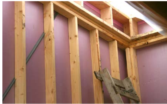
Figure 8: Rigid foam insulation system used in Winnipeg trial home to replace exterior wood sheathing as well as the air barrier, 2015. Photo credit: Gary Proskiw
