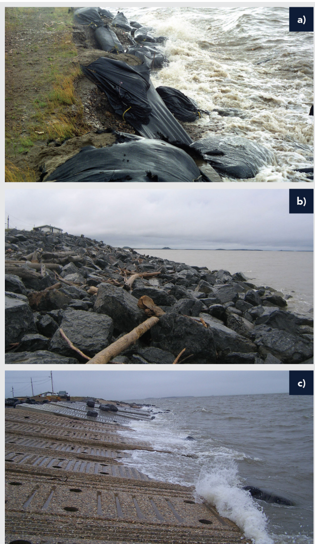
FIGURE 23: Various types of shore-protection measures include a) sandbags put in place in 1987, b) stone boulders (rip-rap) first used in 1997, and c) monolithic concrete slabs that were installed in 1998. Photos a) and b) courtesy of S. Solomon, and photo c) courtesy of G. Manson.
