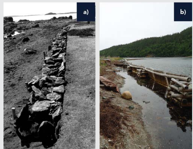
FIGURE 16: Two different construction methods used to protect archeological sites in Bonavista Bay, NL: a) the stone gabion wall constructed at Inspector Island (Pastore, 1987) has successfully protected the site for three decades; b) wooden breakwaters have consistently failed at the Beaches site. Photo b) courtesy of Anita Johnson-Henke.
