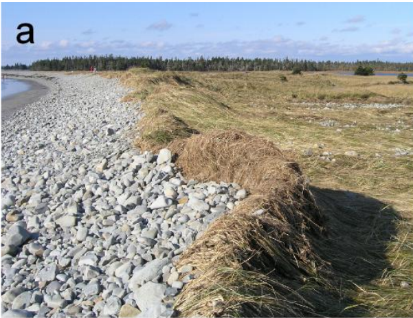
Figure 44. Waves from Noel (a) rolled back the seaward edge of the dune as cobble was pushed higher upslope and (b) transported flotsam and pebble cobble material as much as 75 m into the backshore as shown just east of cross-shore line 1 (marked by pink flags and t-bar circled) . (photos PB090615 and PB090607, Nov. 9, R. Taylor ).
