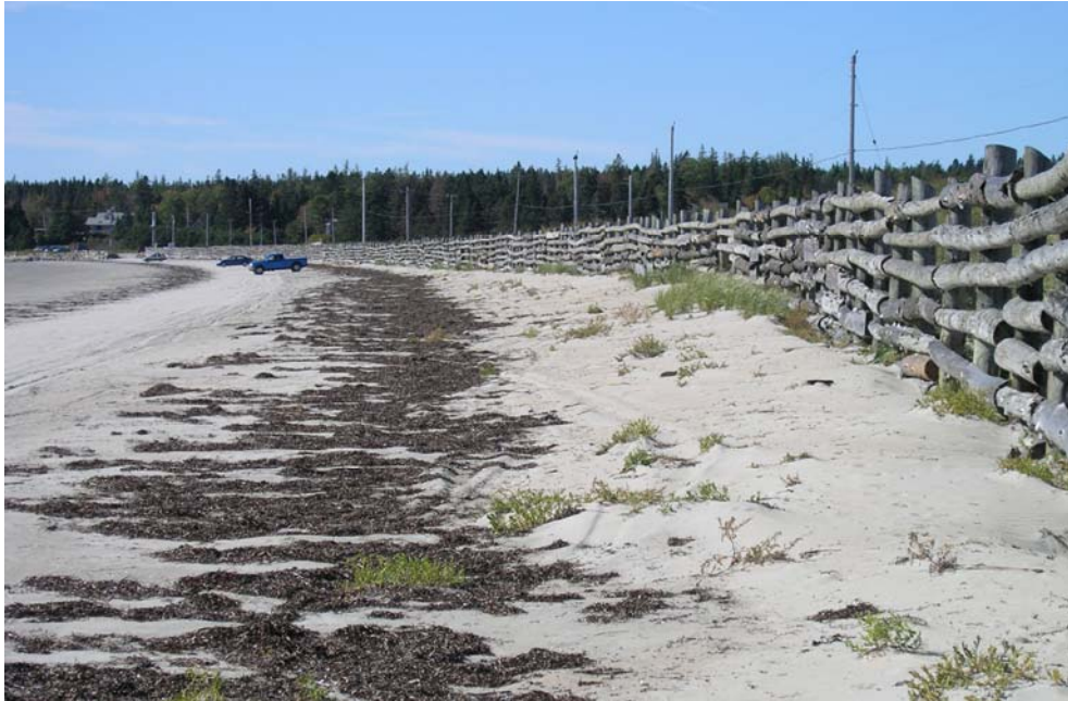
Figure 34. By early October 2007 sand had accumulated along parts of the seaward side of the wooden fence forming a small foredune similar to what had occurred in September 2003 just prior to Hurricane Juan (photo PA070198, R. Taylor)
