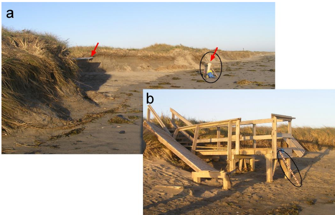
Figure 26. Damage to boardwalks on Martinique Beach varied depending upon their location and condition of beach prior to the storm (a) complete loss of platform (between arrows) between supports and severe scouring of adjacent dunes and b) tossing of access ramp against main boardwalk and steps into the dunes at parking area 8. Most large pieces of boardwalk broken away were carried toward the east end of the beach. A 1.5m long survey pole (circled) is provided for scale in each photo (photos PB040292 and PB040310, Nov. 4, 2007, R.Taylor).
