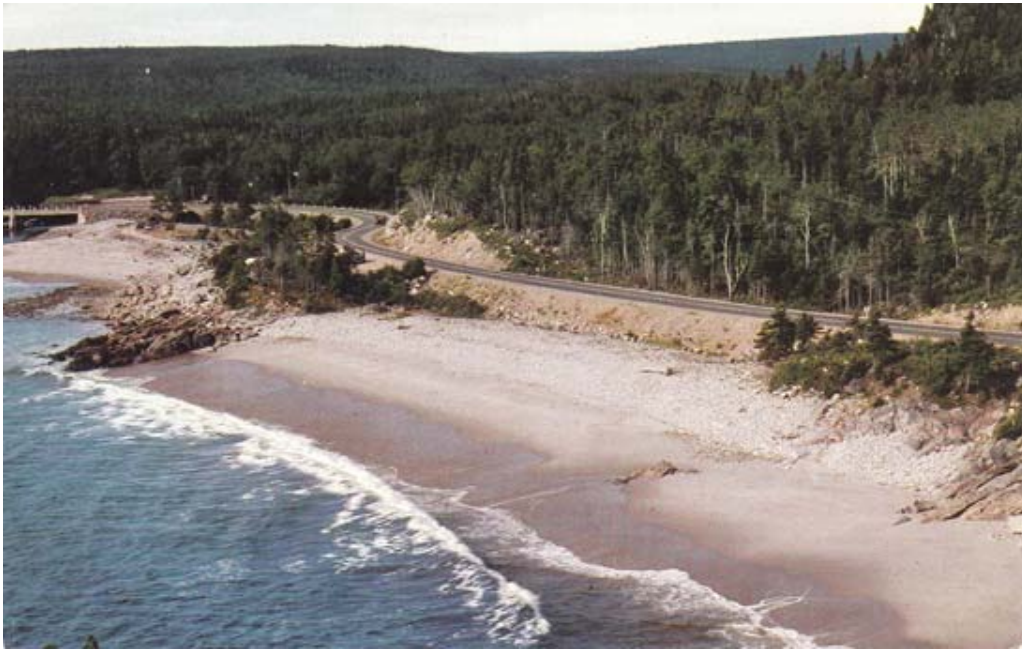
Figure 34. Postcard showing Black Brook Cove Beach in the 1950s (postmarked 1957). A wide sand foreshore and pebble cobble upper beach fringed the coastal highway which was built along the back of the natural backshore. After the road was moved landward in the early 1970s, the former road was widened into a parking area and grass was laid across the backshore (see Fig 3b).
