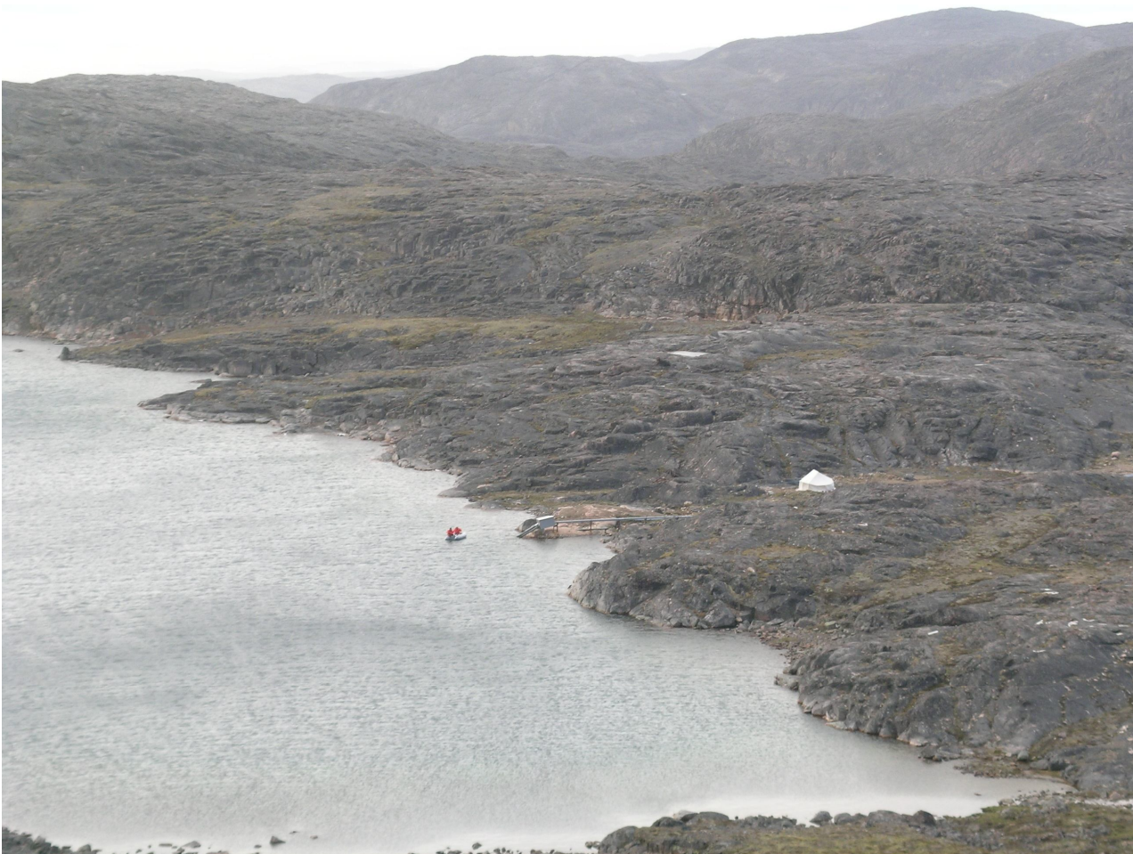
Acquiring underwater video camera footage at T-Lake intake pipe.
