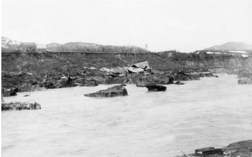
Fig. 2-24. Contemporary post-failure view across the Liève River channel into the landslide scar, showing spoil and destroyed buildings within the landslide crater. The river is flowing from right to left. (Photograph: Archives Nationales du Québec)
