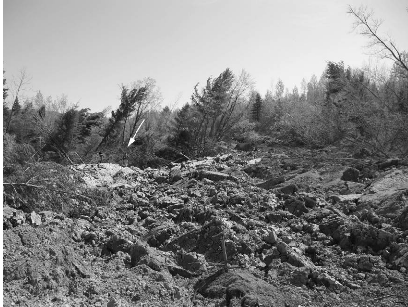
Figure 2-11. Photograph of the 2008 failure taken in early May 2008 showing the fractured Champlain Sea sediments that form the surface of the spoil. Note, the leaning trees in the background that have been rafted by the failure. An arrow marks the location of a person for scale. (Photograph: Gaétan Lessard, Ministère de la sécurité publique du Québec)
