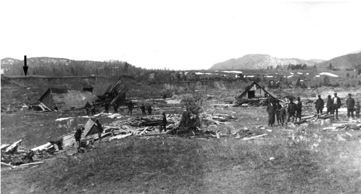
Fig. 2-25 Damaged and destroyed houses within the village of Notre-Dame-de-la-Salette showing the effects of the landslide-generated displacement wave and ice on wooden structures located on the east bank of the Liève River. Arrow marks the headscarp of the landslide. (Photograph: Archives Nationales du Québec)
