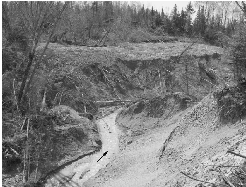
Figure 2-10. Photograph of the incised creek course through the spoil of the 2008 failure, taken in early May 2010. On the surface behind the stream course, note, the weathered appearance to the spoil compared to that shown in Fig. 2-11.
